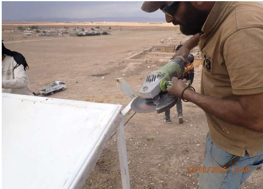
Figure 17: Image showing the cutting of the iron rod that prevented the cover from lying flat
