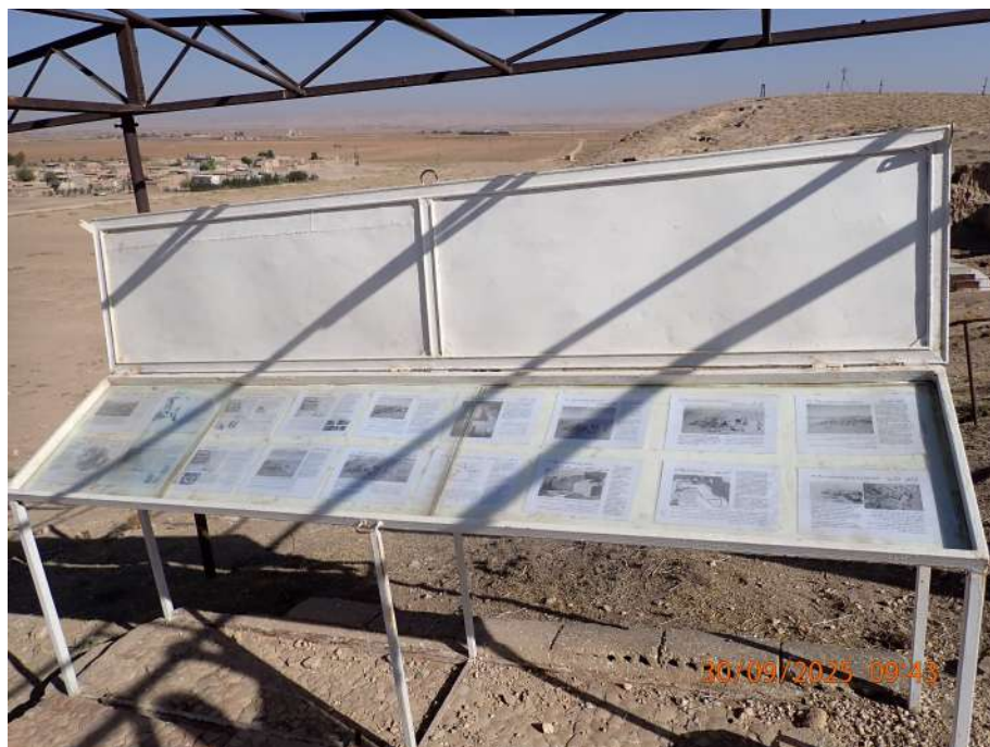
Figure 16: Image showing the cover not resting flat on its base
