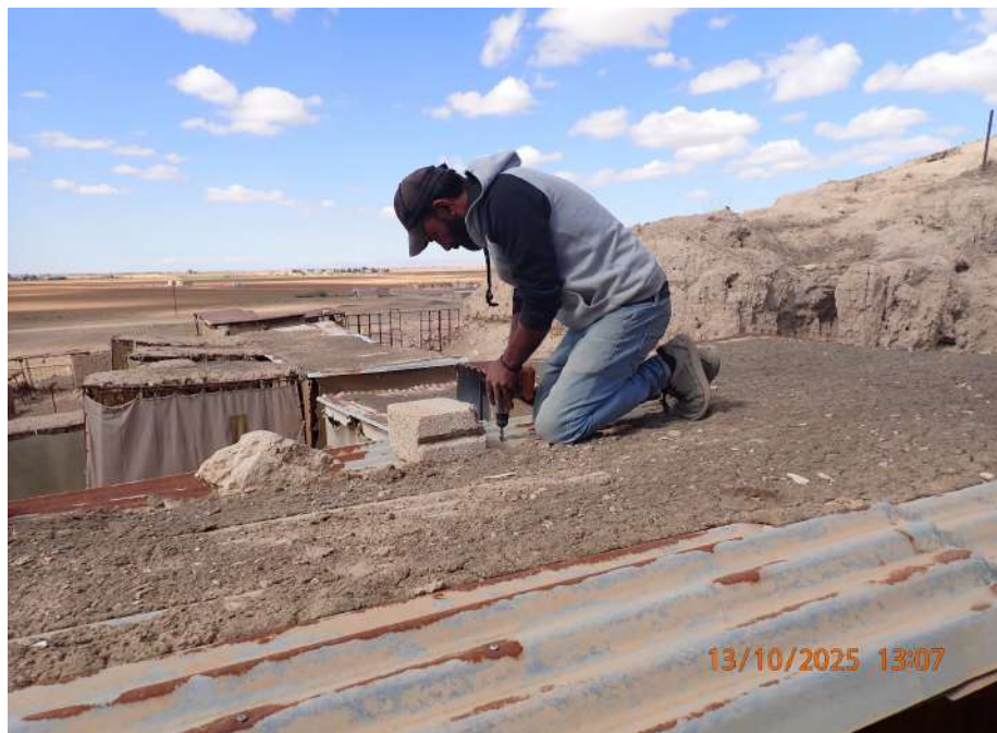
Figure 22: Image showing the securing of the tutiya sheets on Wall D1-I
