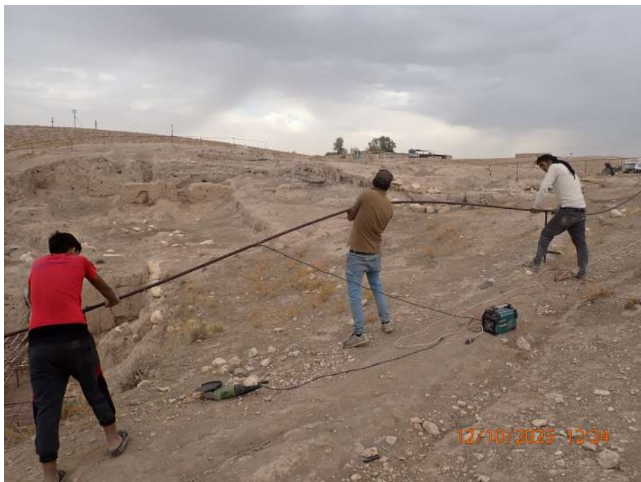
Figure 8: Image showing the straightening of bent rods
