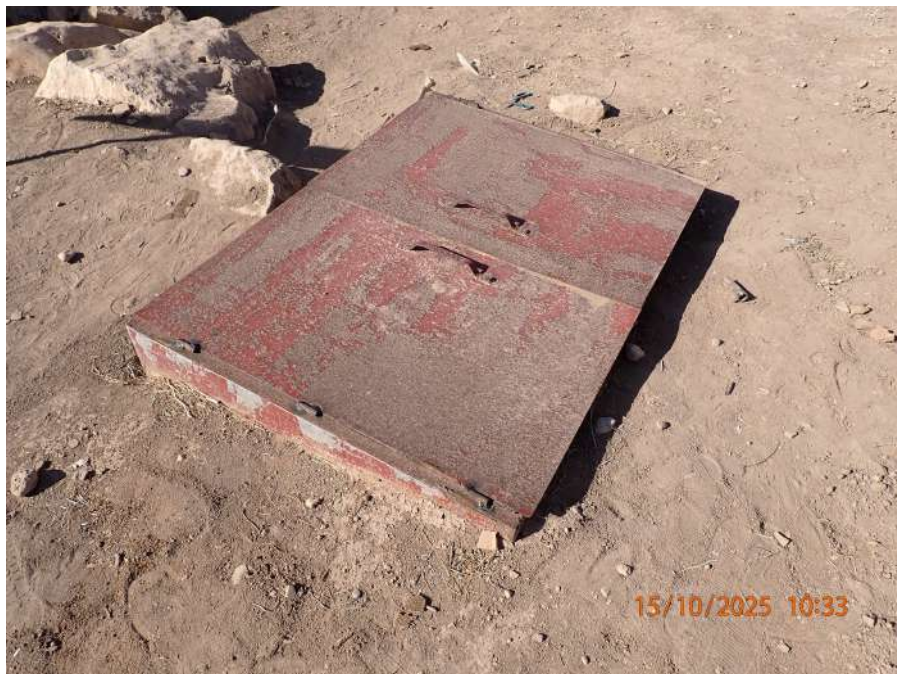
Figure 14: Image showing the tannur cover after repair
