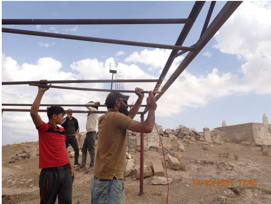
Figure 19: Image showing the repair of the broken canopy above the palace panorama
