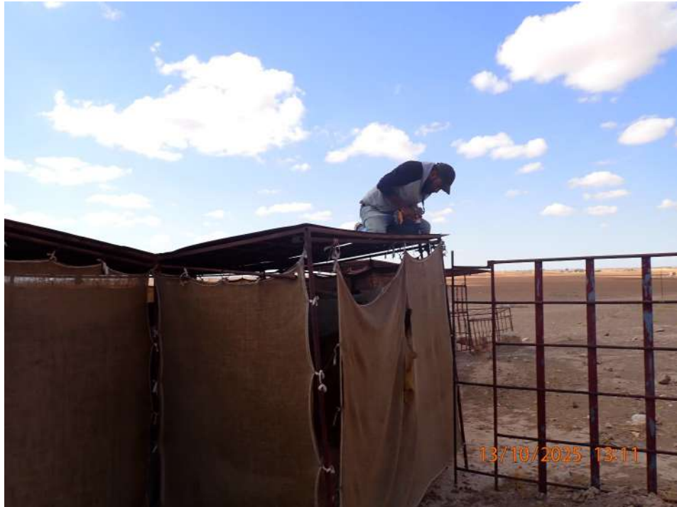
Figure 23: Image showing the securing of the tutiya sheets on Wall E1
