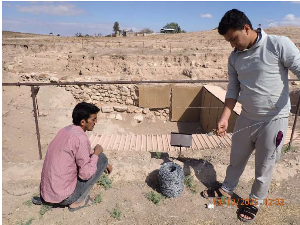
Figure 26: Image showing the reinstalling of the new protective barbed wire
