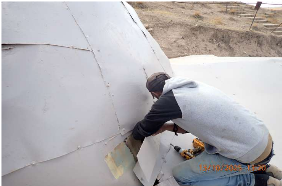
Figure 24: Image showing the re-installation of a missing bolt on the Abi dome
