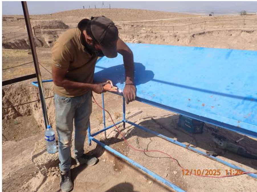
Figure 11: Image showing welding of minor cracks in the temple panorama
