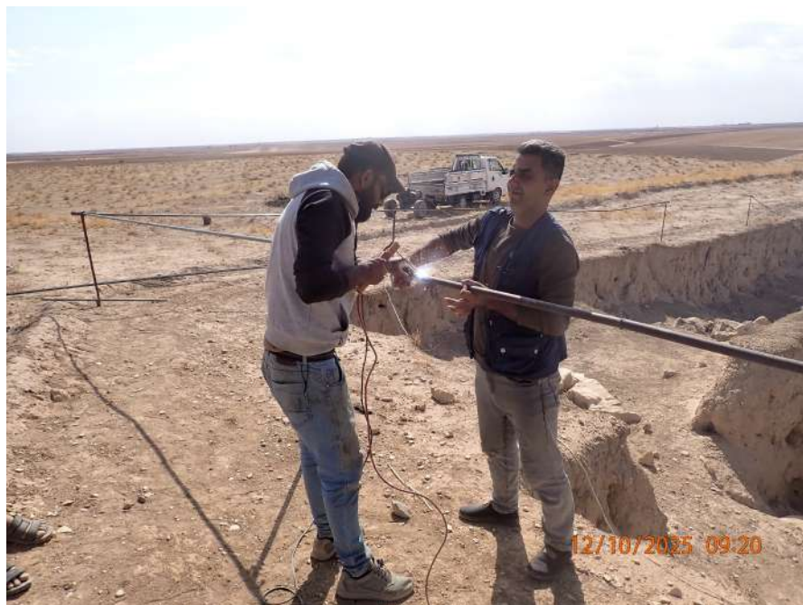
Figure 4: Image showing welding of the rods
