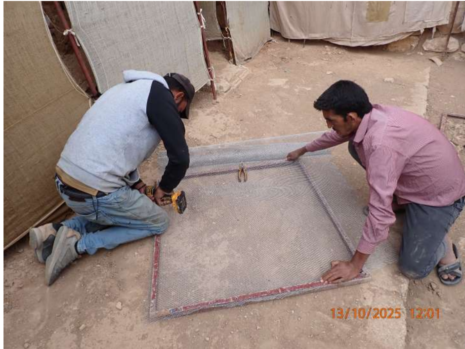
Figure 21: Image showing the installation of the new mesh on the drainage frames
