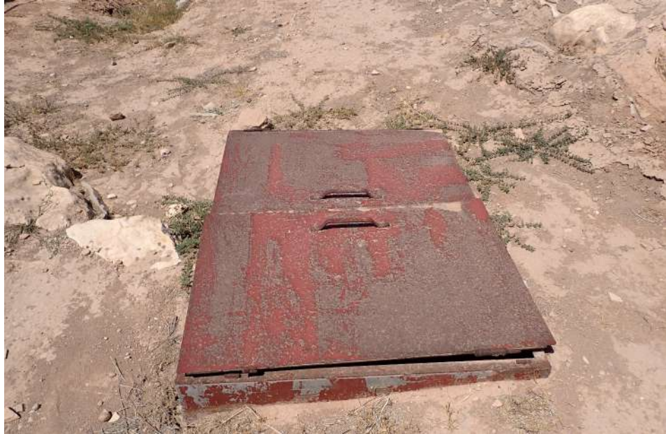
Figure 13: Image showing the broken rings of the tannur cover
