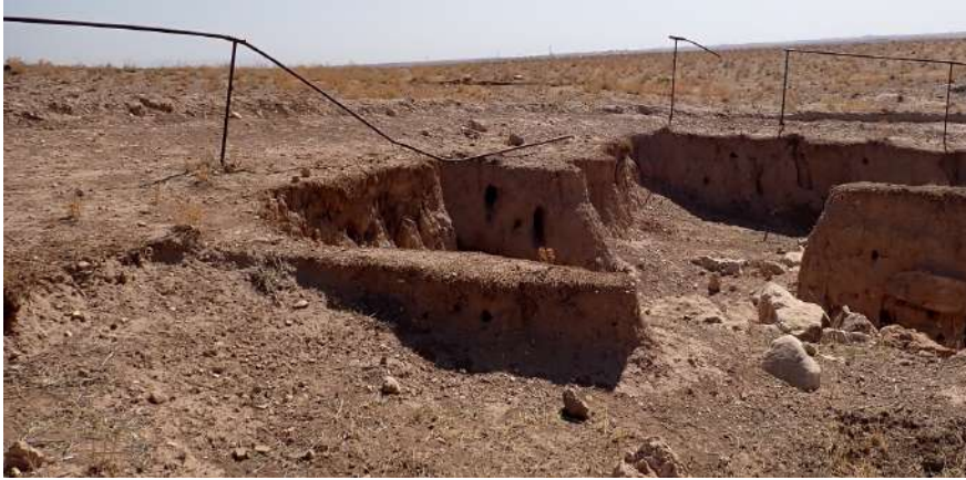
Figure 1: Image showing bent rods
