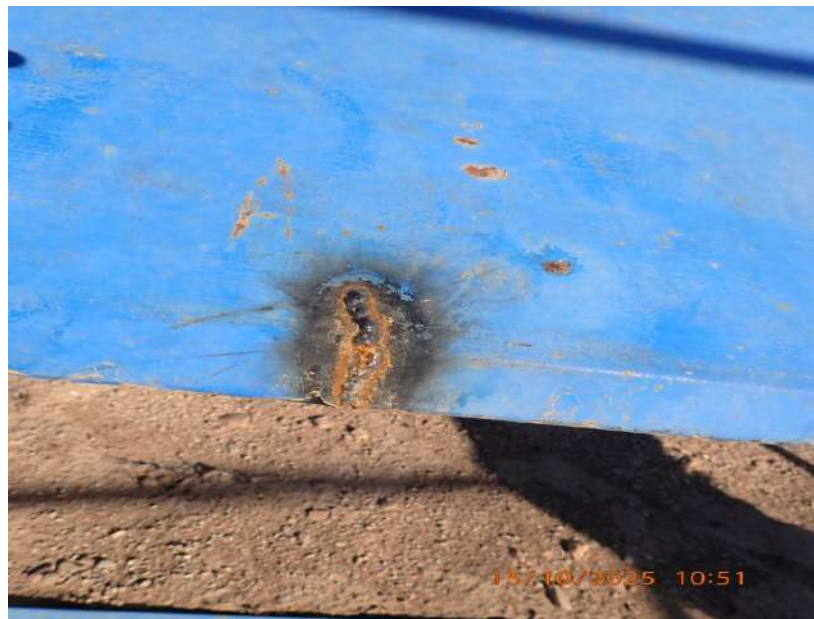
Figure 12: Image showing the panorama after welding
