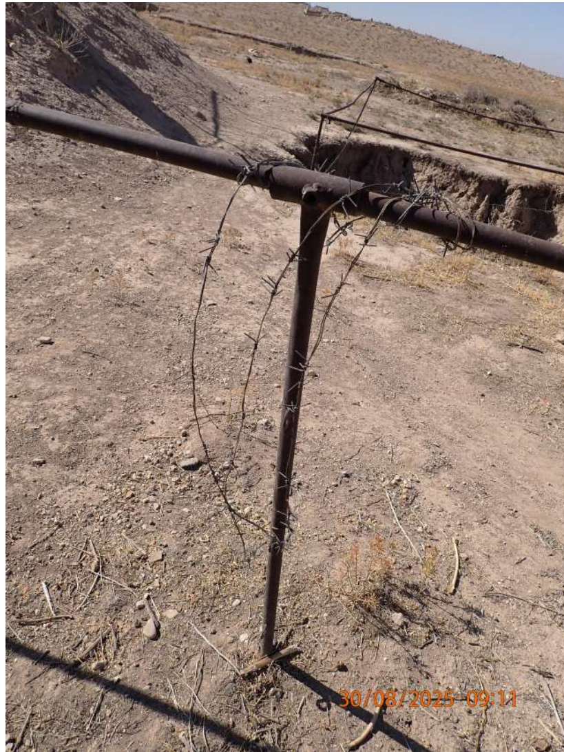
Figure 25: Image showing damaged protective barbed wire
