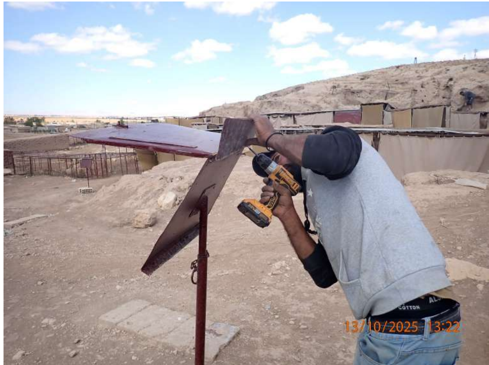
Figure 28: Image showing the installation of screws at the bottom of the Abi panel cover
