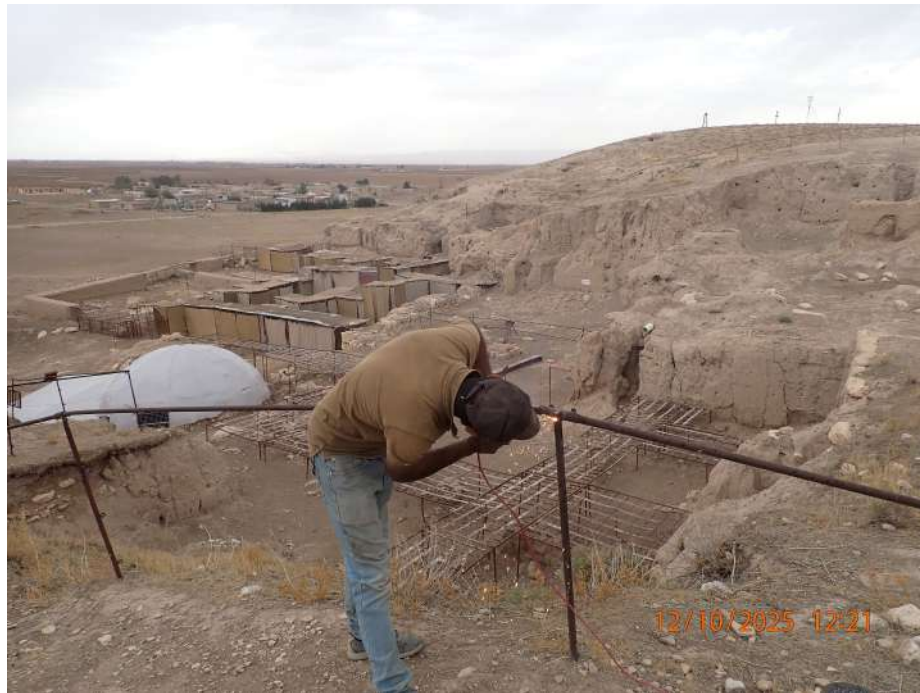
Figure 7: Image showing welding of the rods
