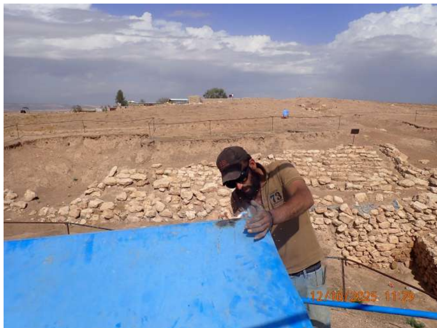
Figure 10: Image showing welding of the panorama corner
