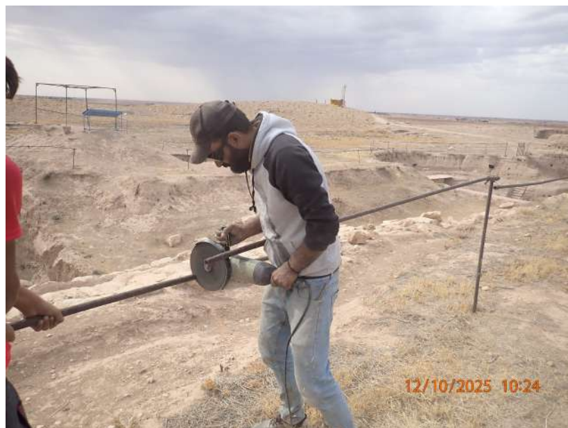
Figure 6: Image showing cutting of parts of the rods
